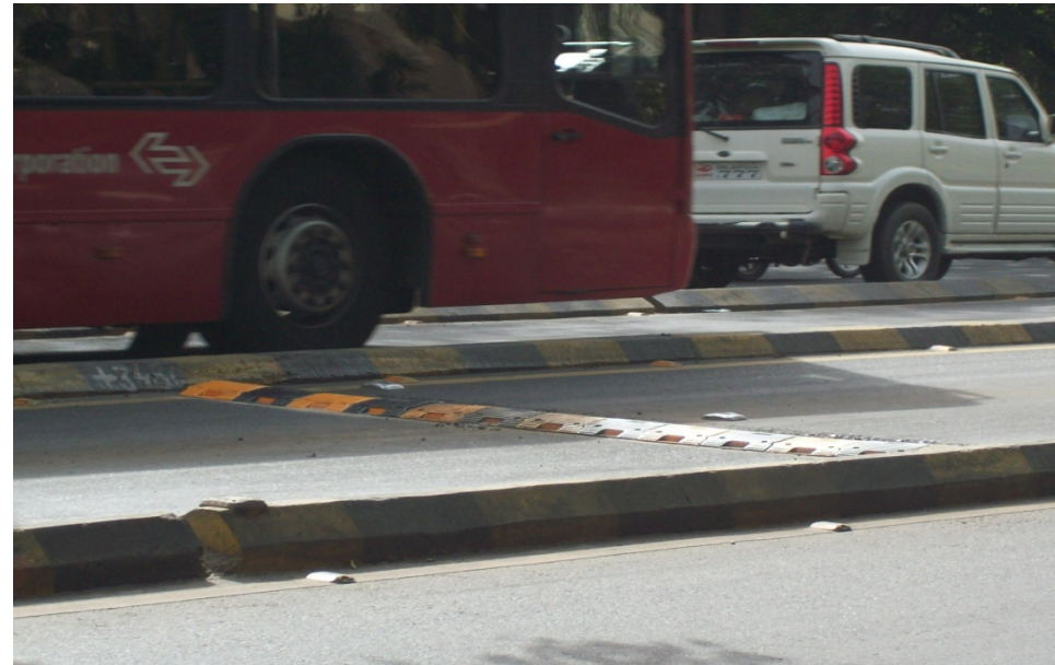
Rumble strip before the bus platform and midblock
